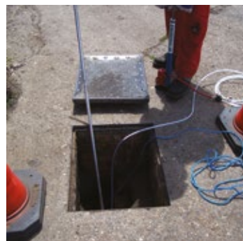
3. Remove lance and disconnect pump
