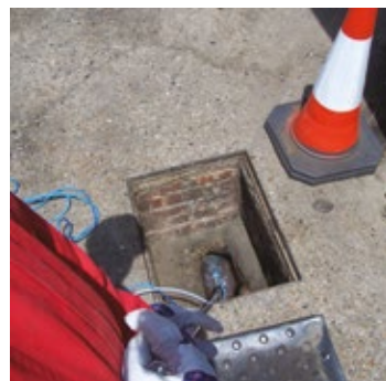
2. Pump up the bladder until fully inflated
