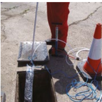
1. Use the lance and rods to insert bladder into drain
