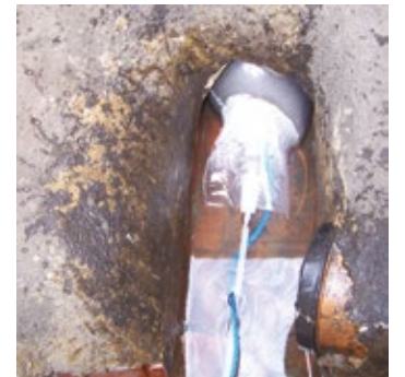
4. Bladder blocking drain
